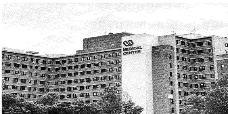
The Veterans Administration hospital near Linwood and Van Brunt boulevards in Kansas City. File photo
